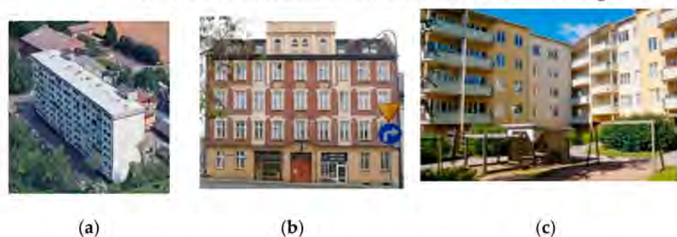
Figure 8. Demonstration sites chosen for the validation of the BIM4EEB developed tools: (a) Italian pilot site; (b) Polish pilot site; (c) Finnish pilot site.
