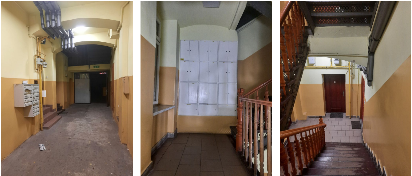
Figure 3 Common space in the Polish pilot building
