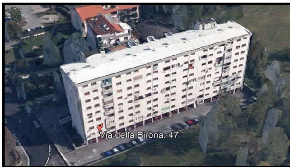
Figure 23: Italian demonstration site
